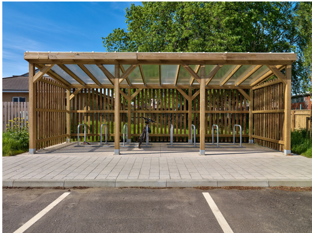
Covered Cycle Storage Area
