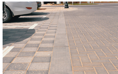
Flush Slipform Concrete Kerb
