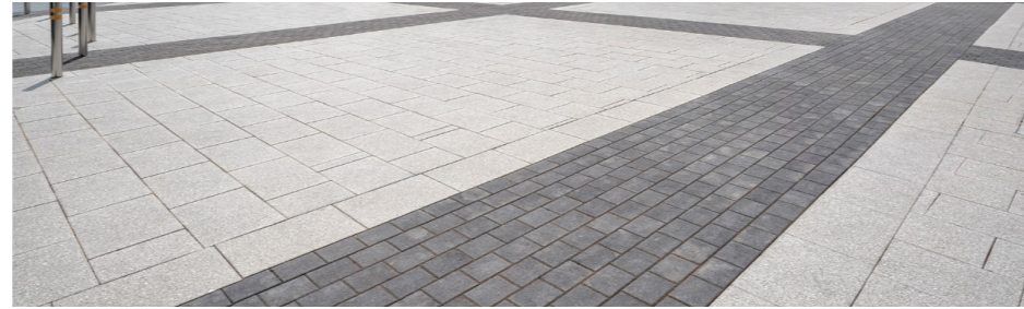
Light coloured flags to maximum light within courtyards w/ contrasting paving blocks
